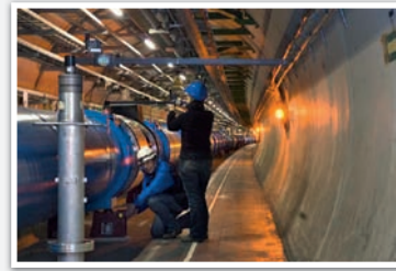
Regular checks are performed to ensure that magnets in the Large Hadron Collider tunnel are perfectly aligned, as they are needed to control the paths of the particle beams.
